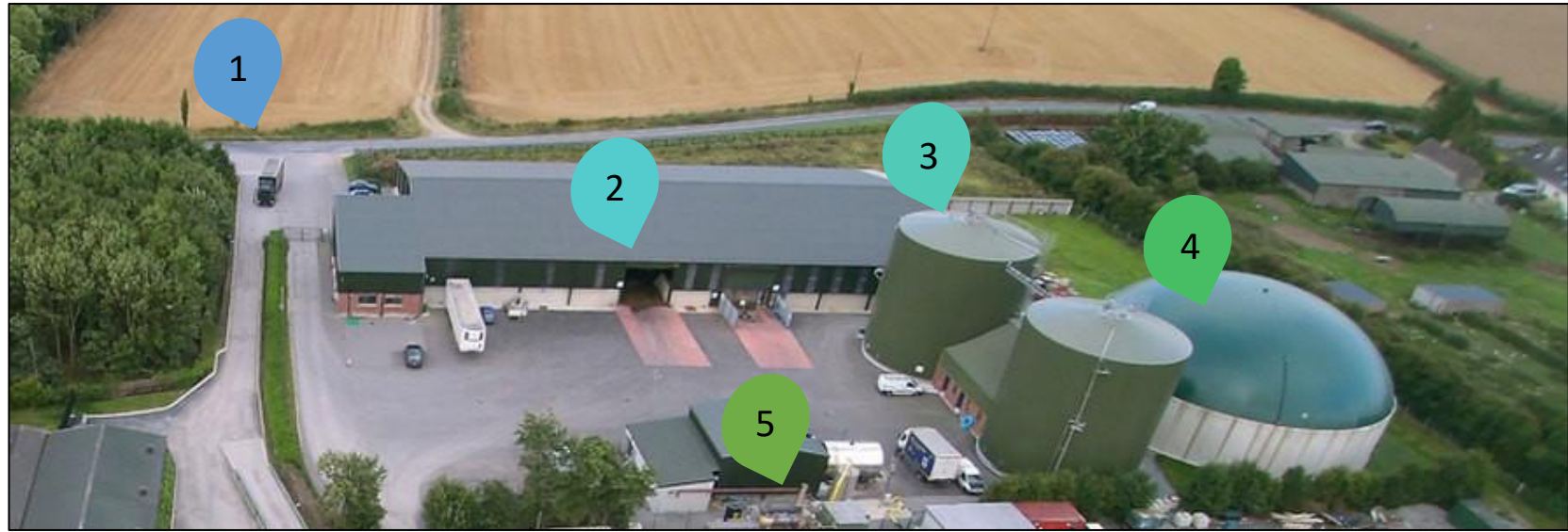
Green Generation AD Plant, Nurney, Co. Kildare.
